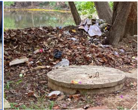
Soak chamber outside Science building for collecting waste
